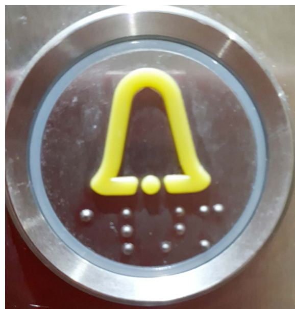
Braille on lift buttons. This one says "alarm".
